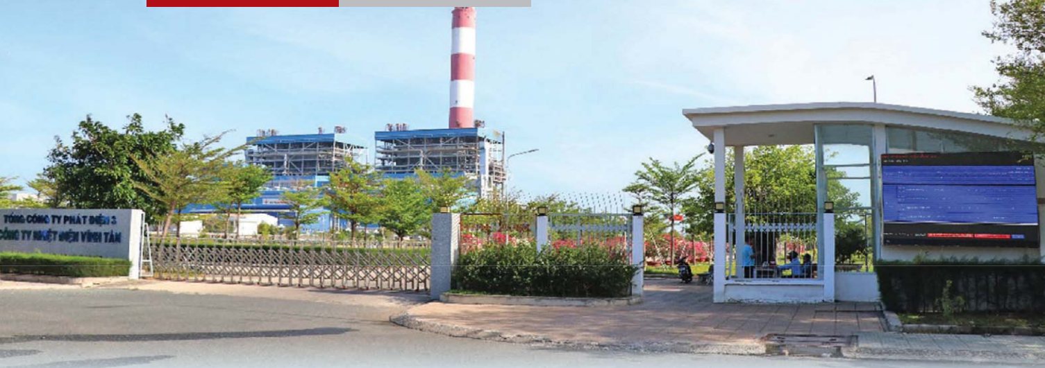
Screen displaying live environmental parameters at Vinh Tan 2 Thermal Power Plant
