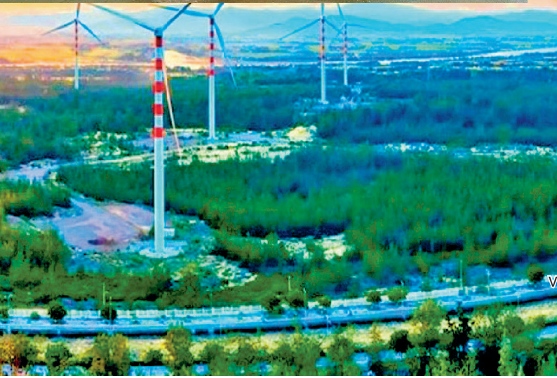
Power generation units operating at la Ly
